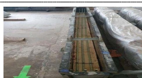
Figure 6. GFRP Bar installation
